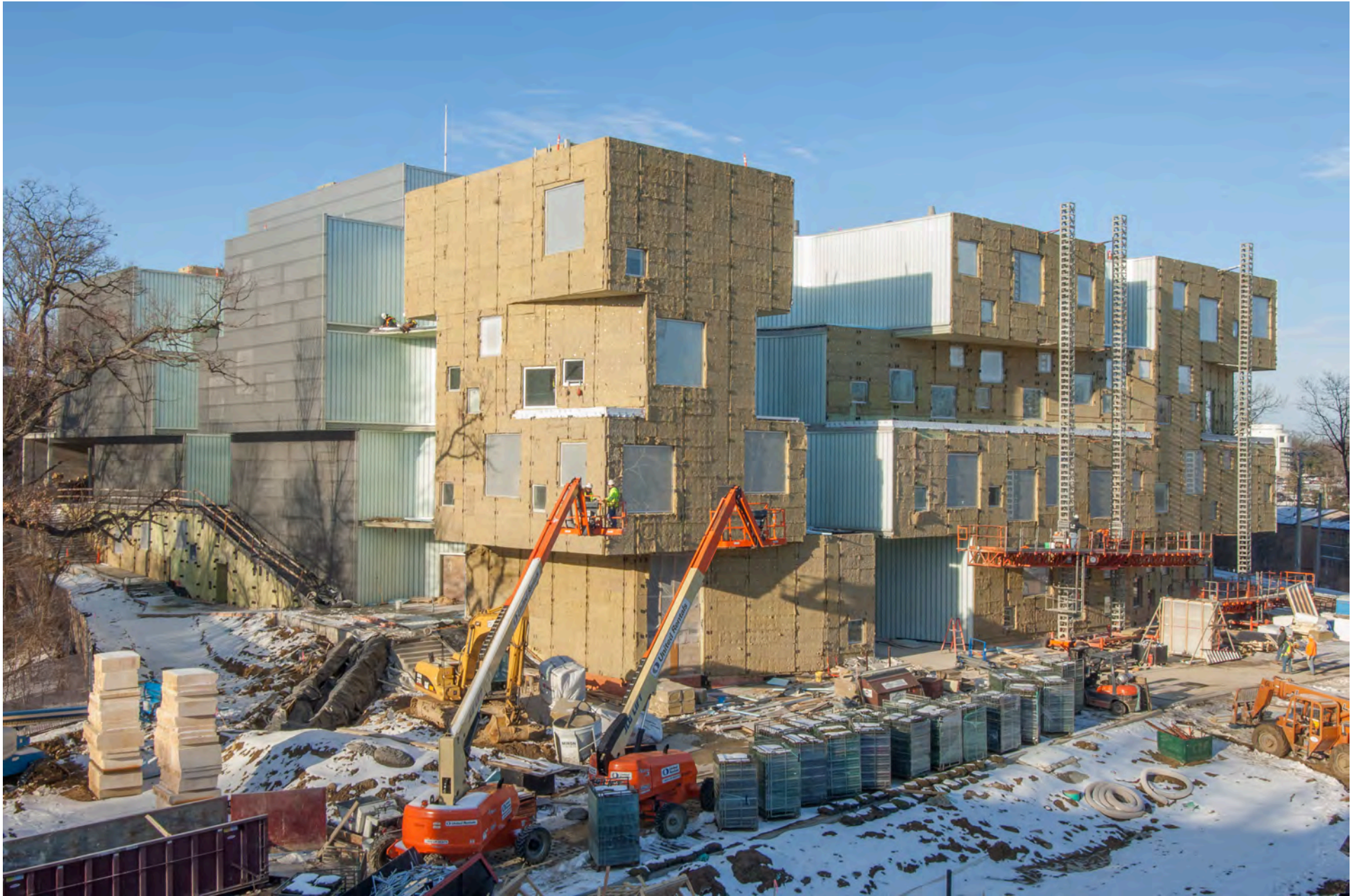
Concrete walls overlaid with thermal insulation and rheinzink cladding mesh
