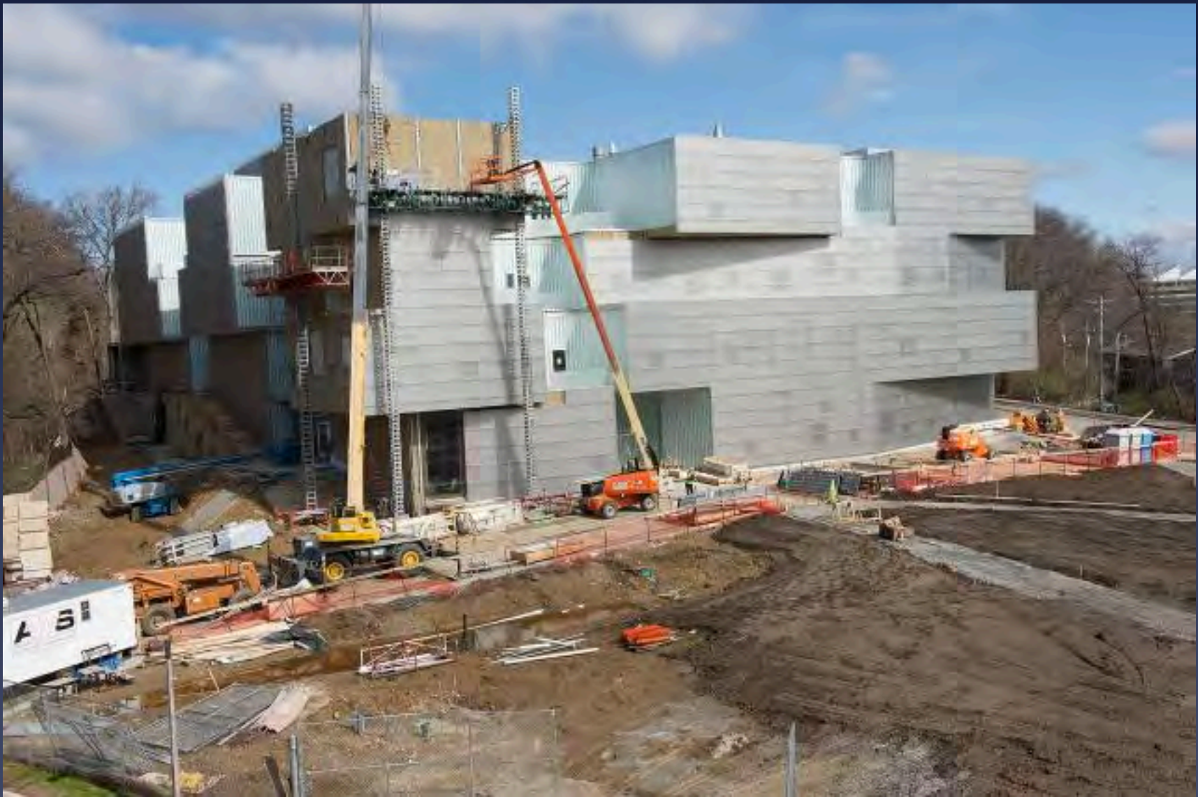
Perforated zinc screen being installed
