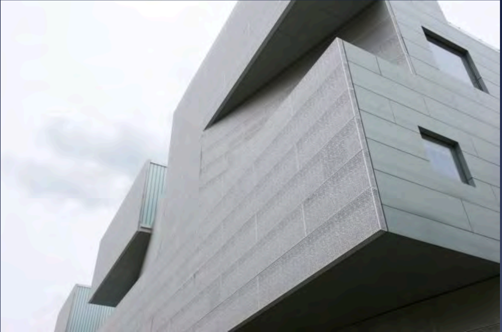
Perforated screen meets flat zinc panel at the corner
