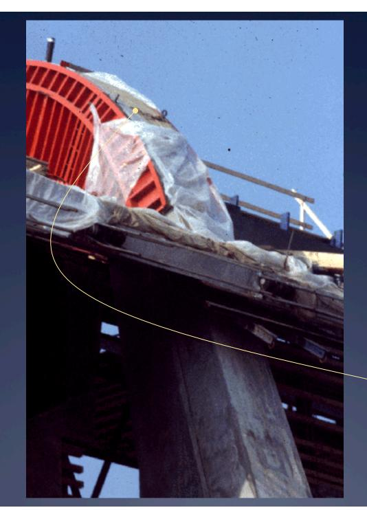
The access doors used to fill the lower part of the top form leak a bit.
