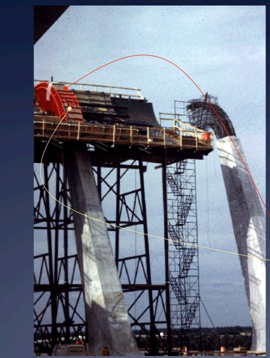
When concrete is poured on sloping surfaces, it needs to be restrained from flowing downhill (especially with plasticizers in the mix)
