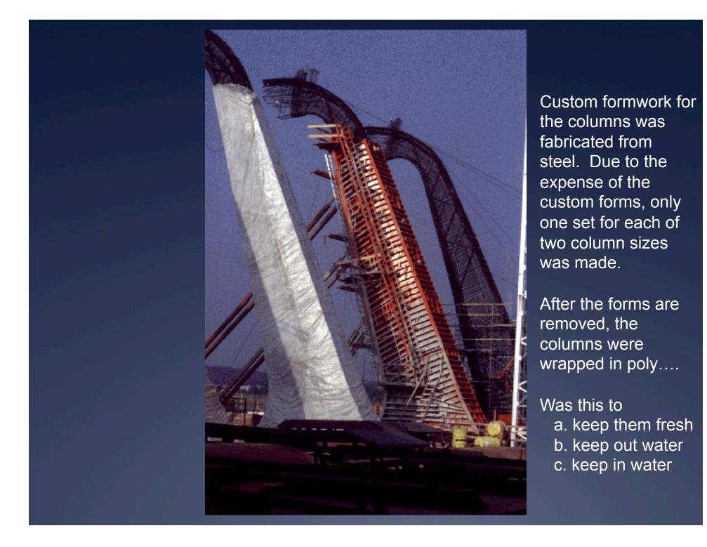
Reinforcing is heaviest at the top and bottom of the column.
