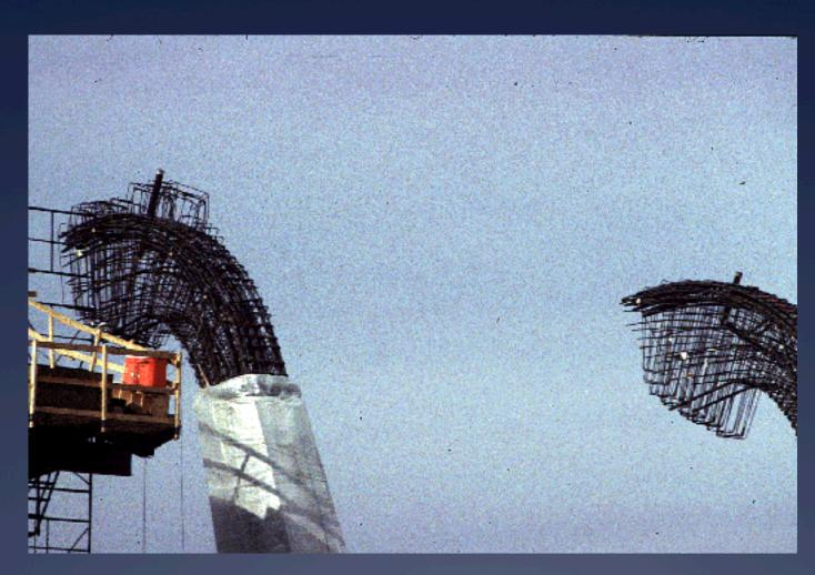
The heavy reinforcing (#18's!) from the top and bottom of the column converge at the column head where it will ultimately connect to the curved roof edge beam.
