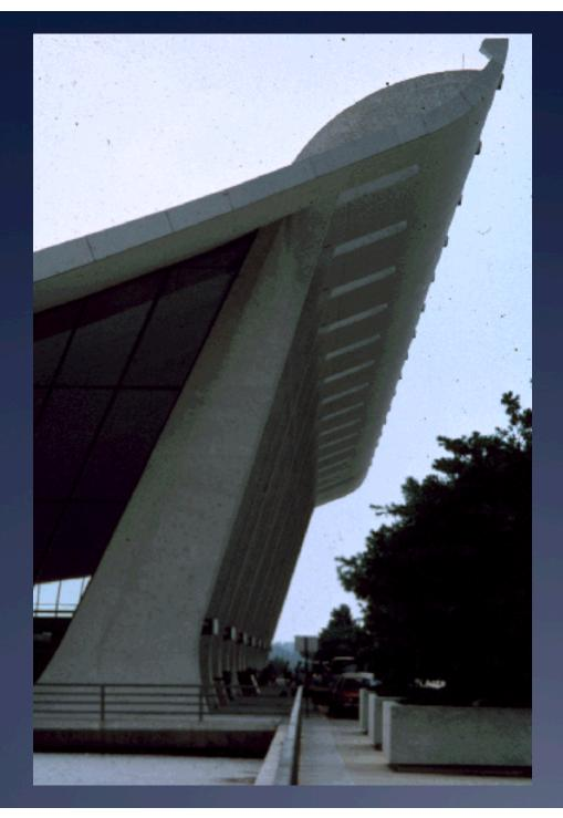
Saarinen's terminal is a landmark building in sitecast concrete. The fluid nature of concrete makes the expressive columns and roof possible.
