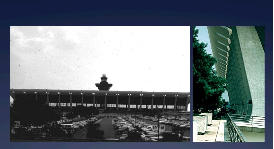
Eero Saarinen had a simple pallette of elements in this project, two columns and a curved roof. Very similar to the Lyon TGV station by Santiago Callatrava, Dulles Airport Terminal uses a very small number of elements repeated a large number of times to make the custom formwork affordable.
