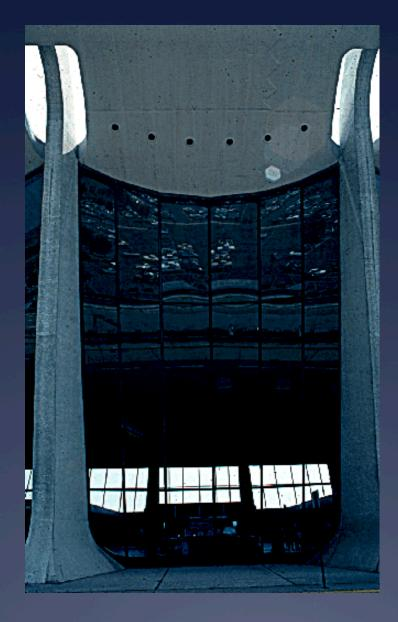
The curtain walls between columns are curved to form a plan shape that is stronger than a flat plane.... Similar to corrugations in cardboard.
