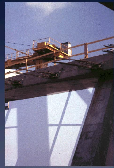
The inside edge of the perimeter beam has heavy reinforcing extending to be tied in to the catenary roof reinforcing.
