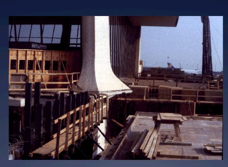
The column's form is termed an 'expression' of the load because below the column is a small pier which carries the column load to the earth. The wider parts of the column are unsupported, part of a structural expression
