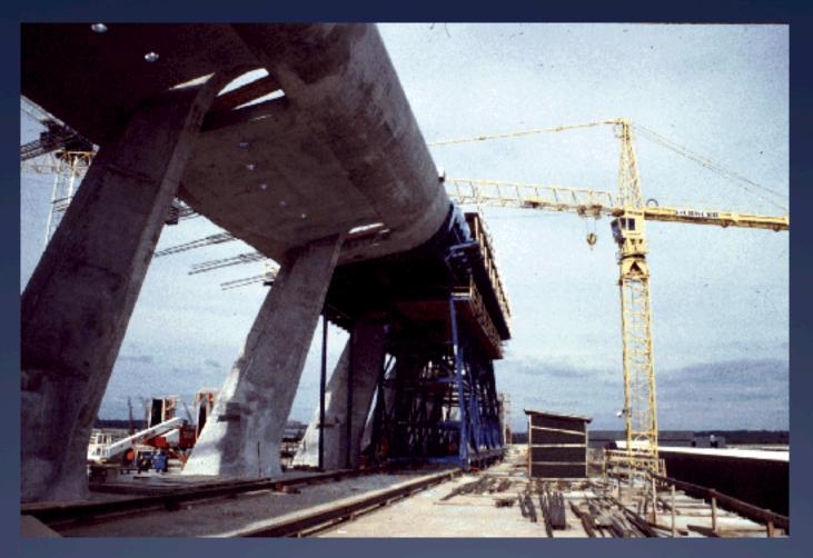
The form is static during the pour. But it is common on high rise elevator cores to have the forms slowly creep vertically during a pour that begins at the footing and doesn't stop until it tops out at the sky. *(Slipforming)*
