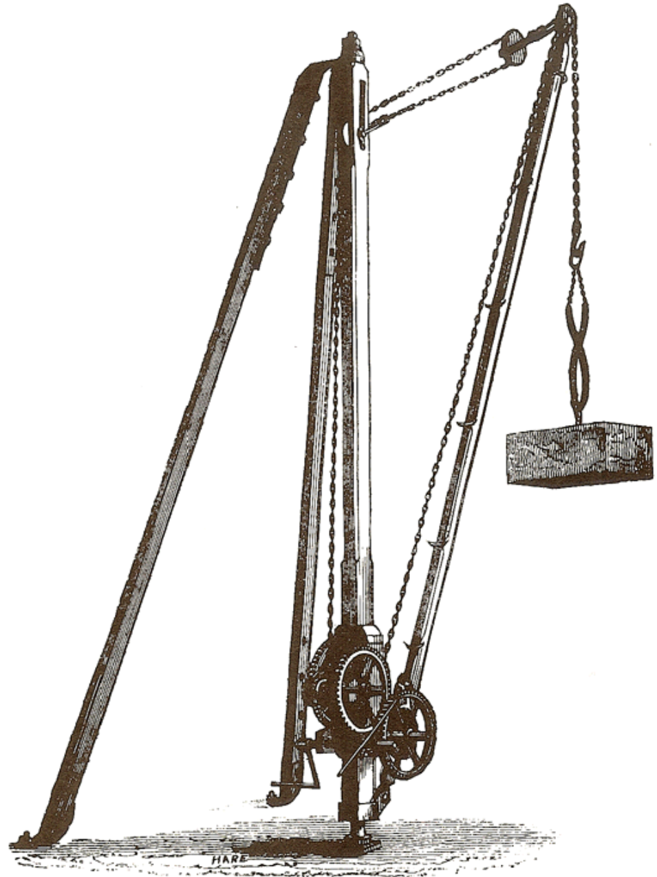
Derrick crane used at Granton Pier (Edinburgh.)
