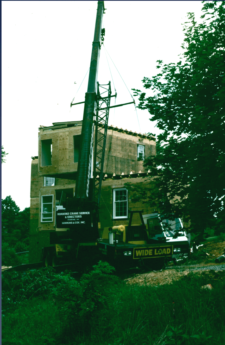
...the crane sets the master bedroom/bath/laundry module
