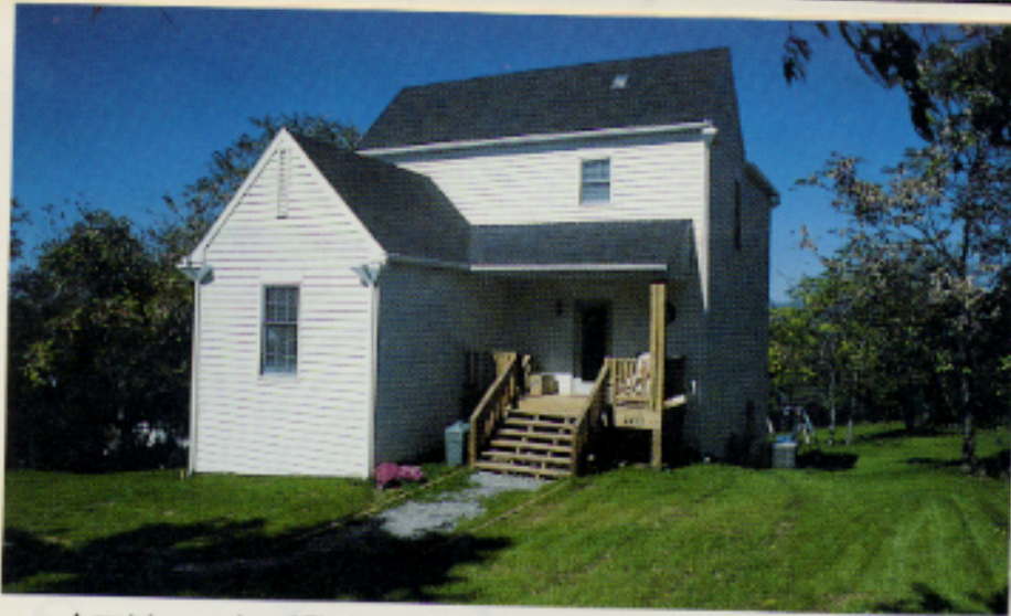
A prototype version of The Maryland, built in Blacksburg, VA, incorporates some additional design touches, three more windows and a few other construction details that added about $500 to the cost.
