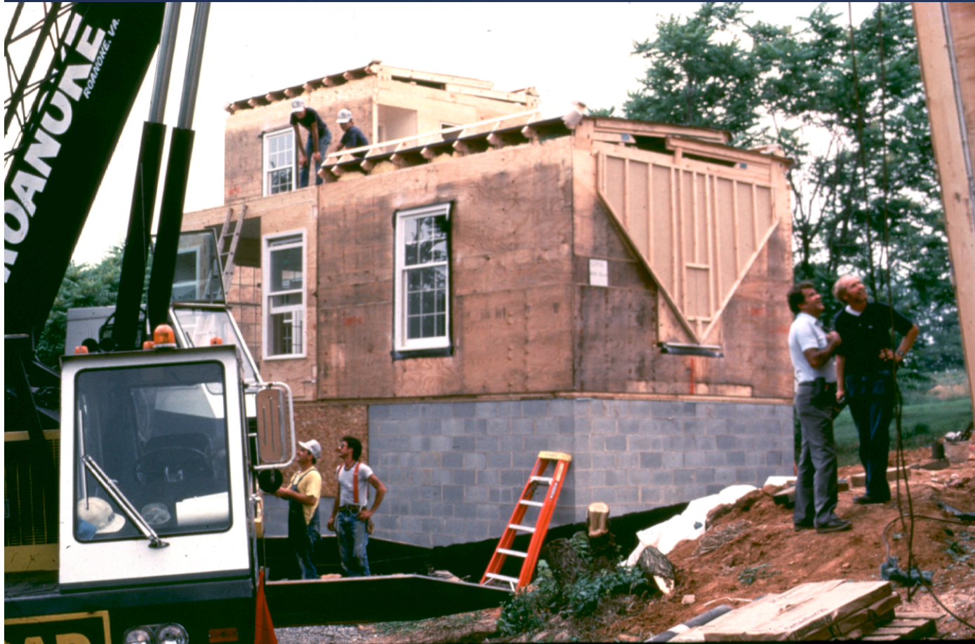
...Donny and Ruk have popped in the living room windows (the ones to the left without the tar paper flashing around them...something we'd have to fix later...)
