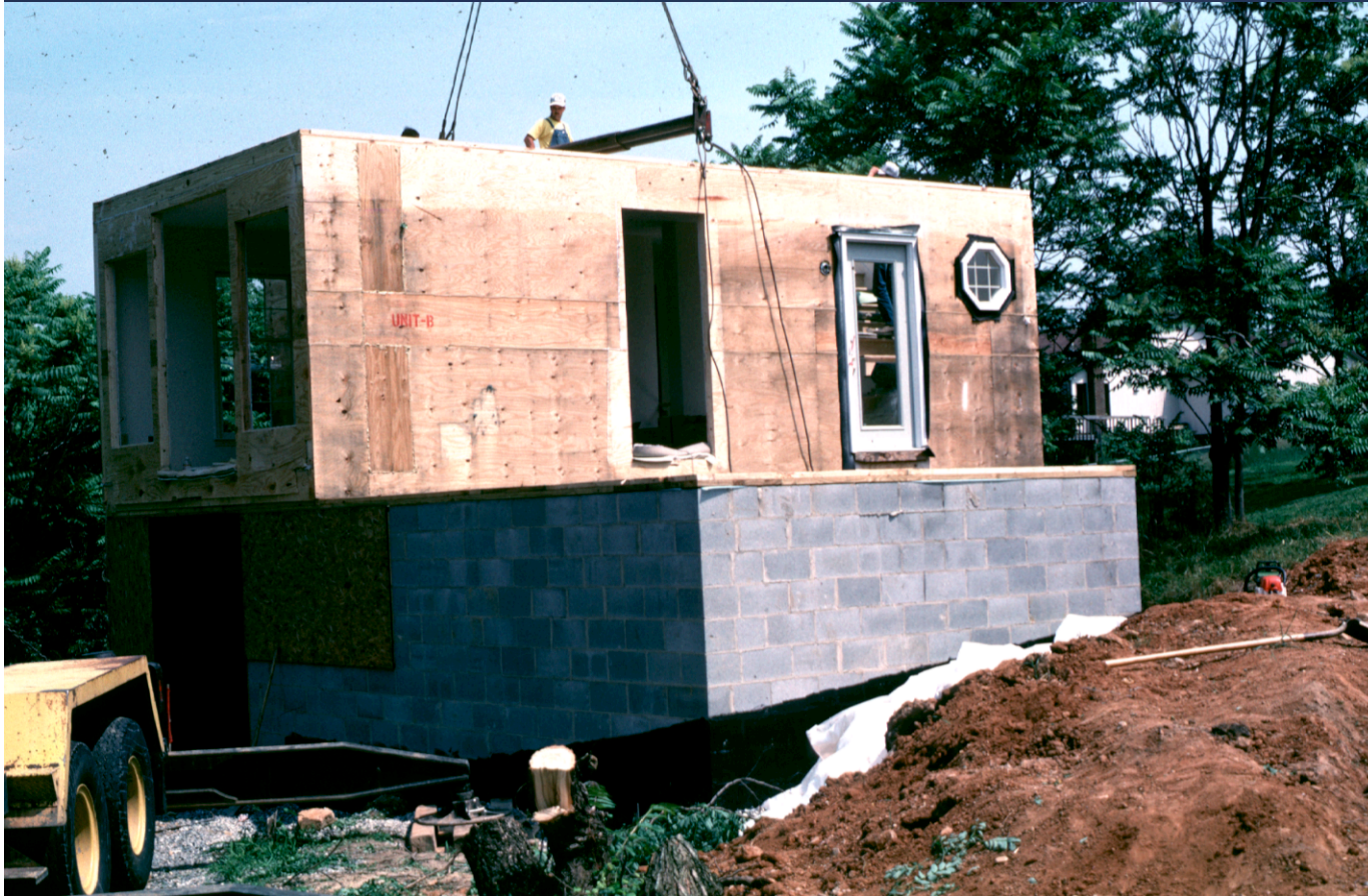
...the crane lifts and sets the completed entry/living room module
