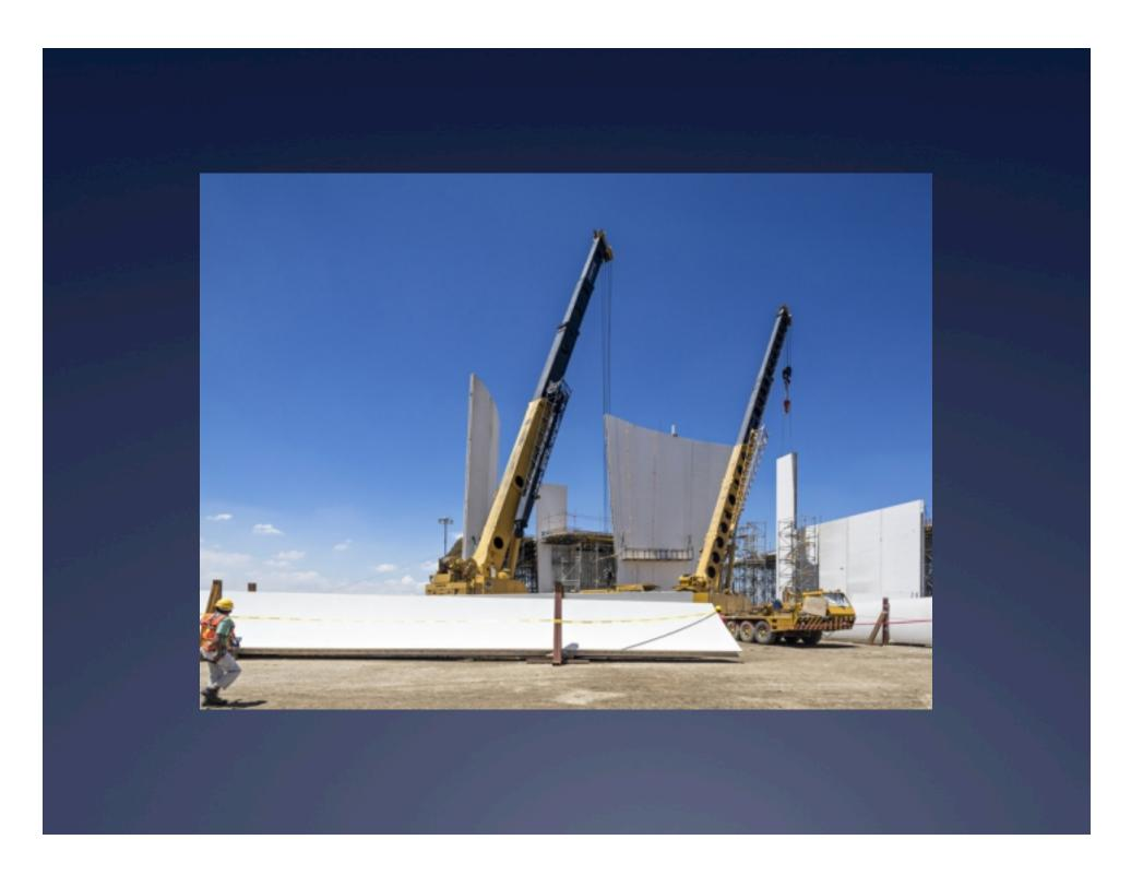
Two panels each 14 inches thick make the formwork... couldn't withstand vibration...had to use selfleveling concrete
