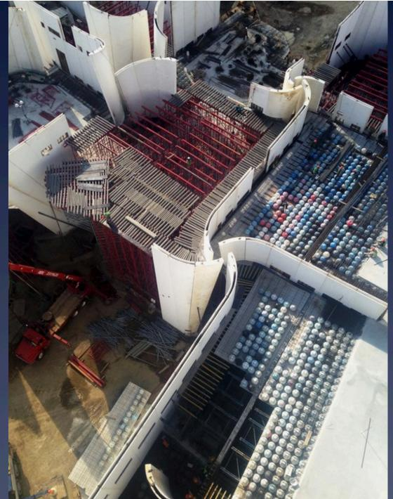
Bubble slab makes the floor lighter to span farther
