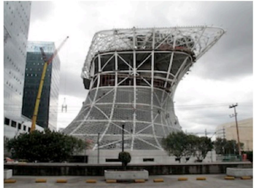
Layer after layer, Geometrica's "spiders" were hung from the main structure rather than set on the floor.
