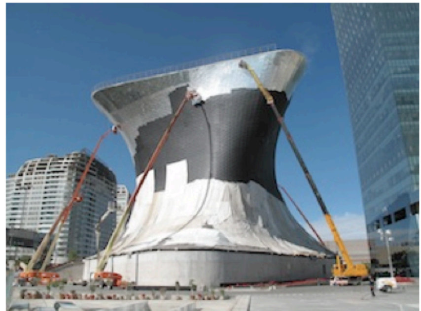
Layer after layer, Geometrica's "spiders" were hung from the main structure rather than set on the floor.
