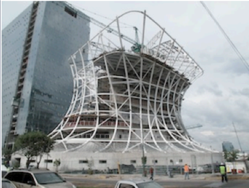
The primary structure was not completed when Geometrica's work began.
