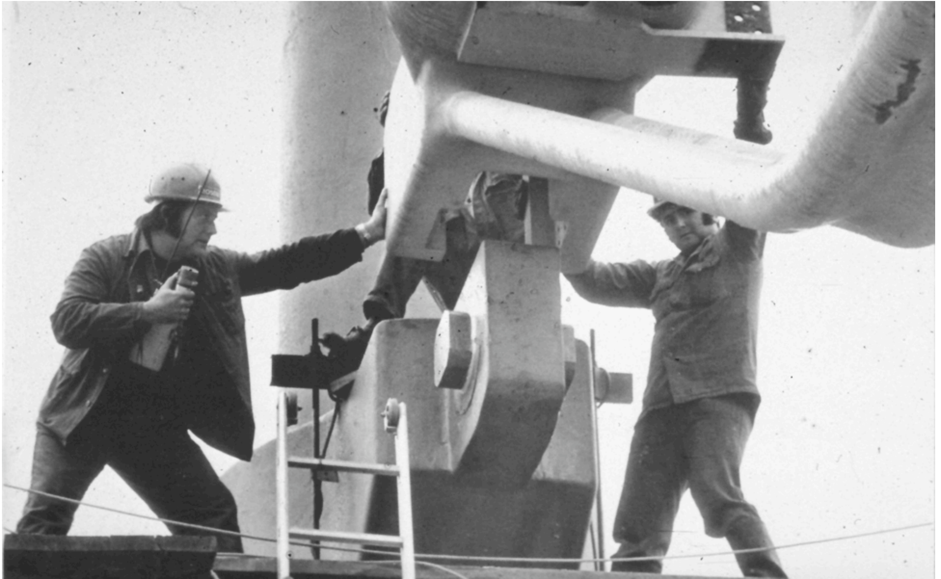
48 meter clear spanning trusses weight down the back of the Gerberettes...believe in gravity
