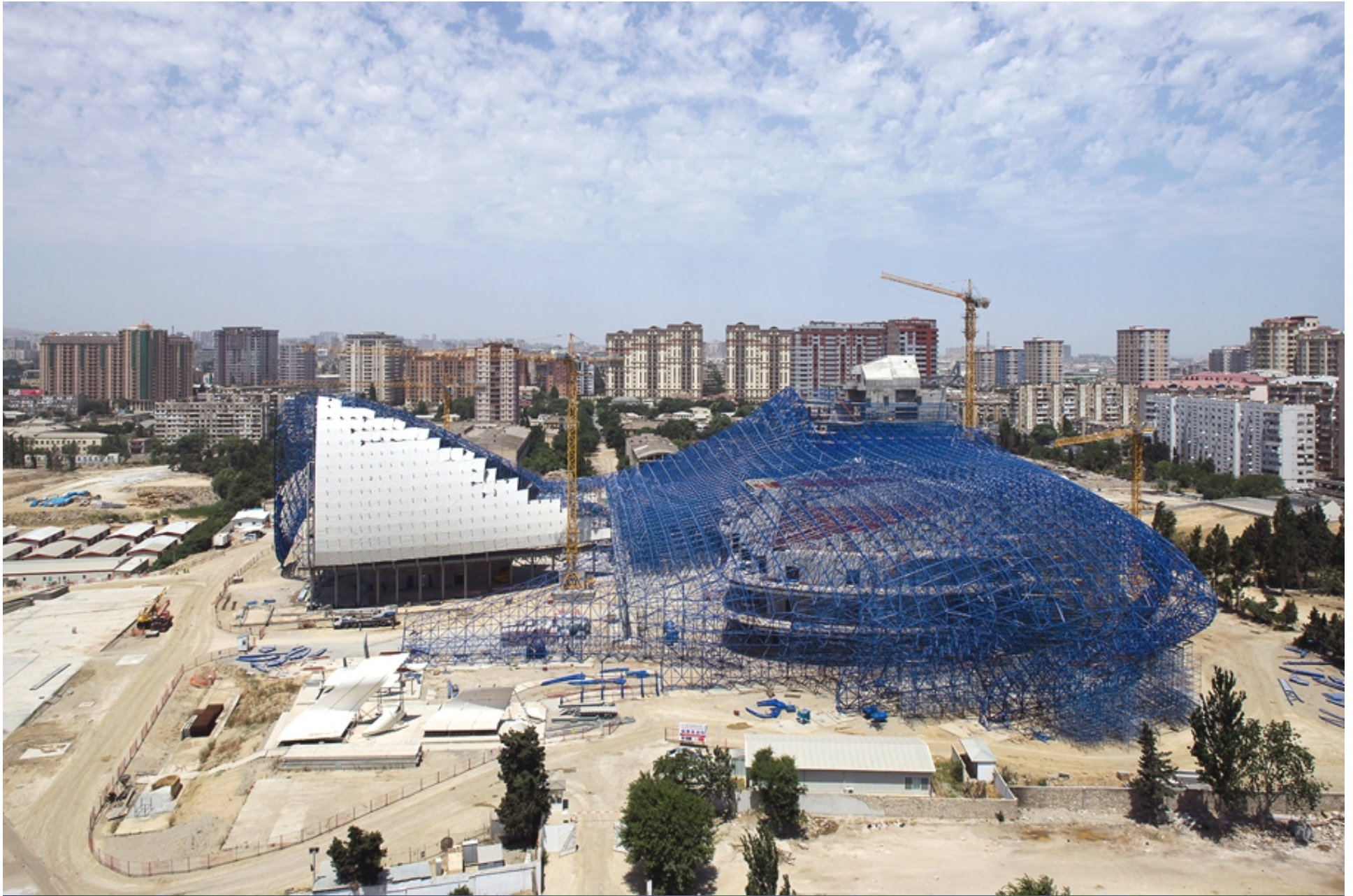
MERO spaceframe, 2,500 tons lighter than alternative trusses
