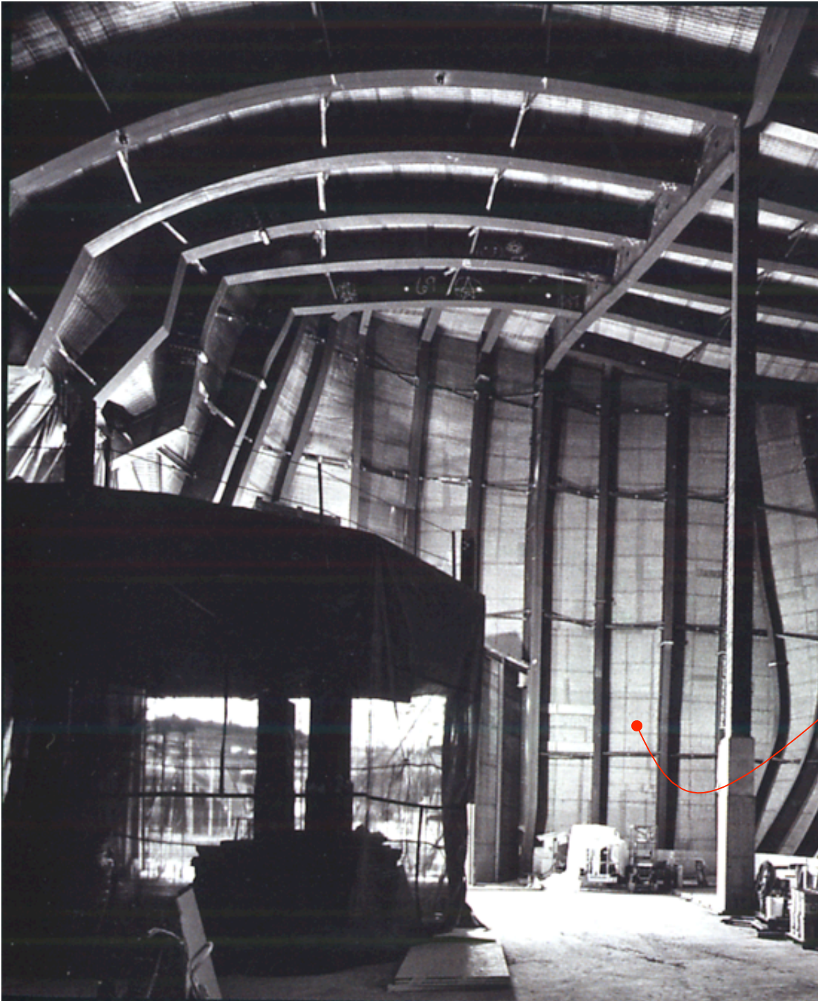
Foil-backed insulation blankets between the steel noodles
