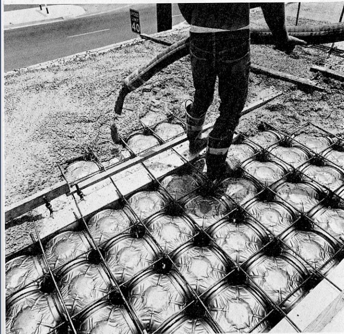
Hollow URBS floors enable ducts to extend in two directions. Ducts are laid on precast concrete bottom slab, arched forms are installed atop stub columns, and top slab is cast on them.
